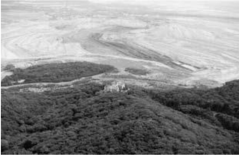
A view from the Ore Mountains of the stabilization pillar below Chateau Jezeří with the arboretum preserved. The coal mine is in the background.
