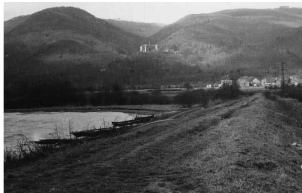
Chateau Jezeří on the Ore Mountains slope above the Dřínov reservoir. Albrechtice to the right. Deep under the reservoir and the village is the coal seam, stretching all the way to the mountainside. Picture taken in 1978, before the opencast mine expanded to this area.
