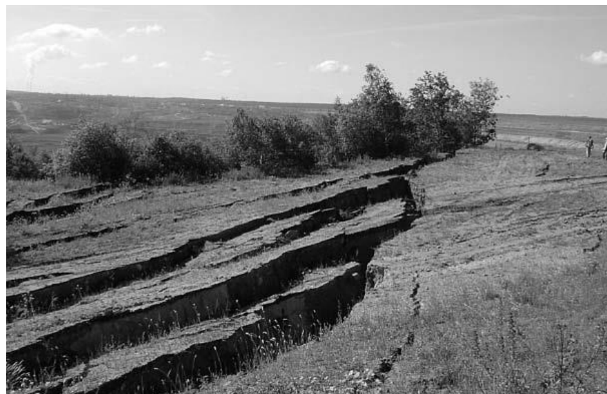
The large-scale open cast mine is a permanent threat to areas beyond the mining limits, as attested by the slide of about 3 million m 3 of earth in the arboretum protective column in June 2005.
