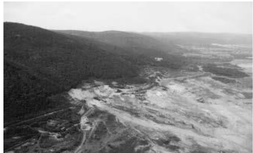
The section of the Ore Mountains side between Jezerka and Jezeří affected by mining in the 1980s. Cutting down the mountainside has caused landslides, which have continued to this day in some places.
